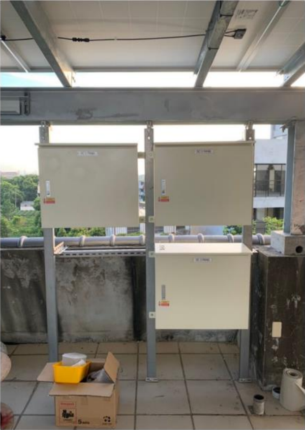
Frame Support (on floor)
