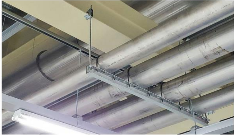
Frame support (From ceiling)
