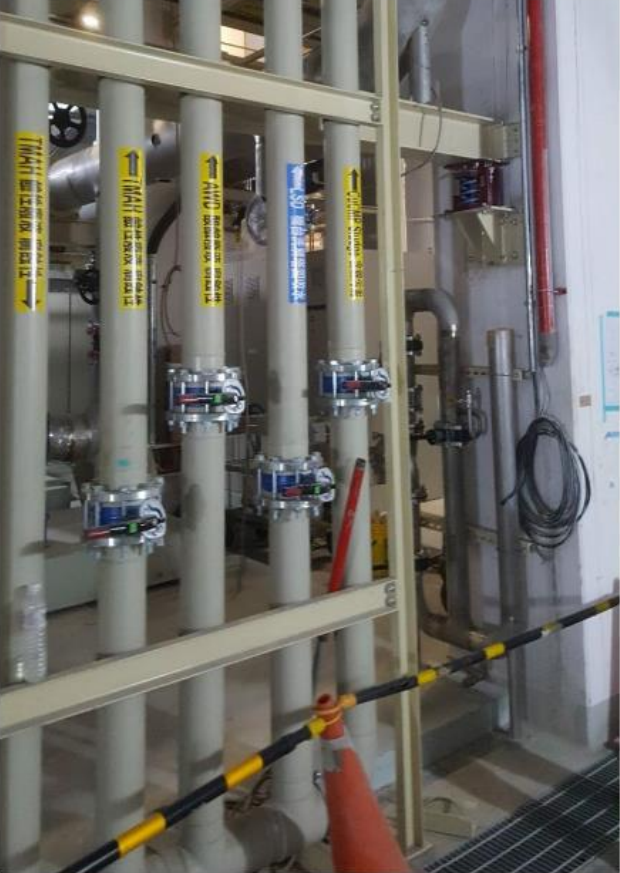
Frame Support (on floor)
