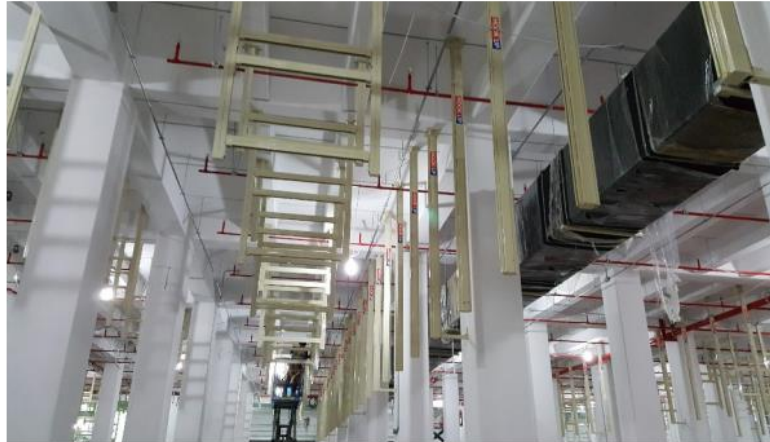
Frame support (From ceiling)
